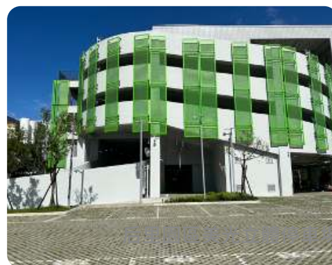
Micron Multi-Story Parking Garage in the Houli Park
