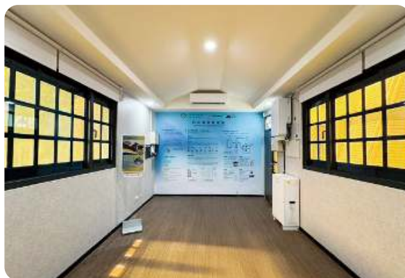
The windows on both sides feature AIZ Windows ZERO perovskite energy-generating windows
