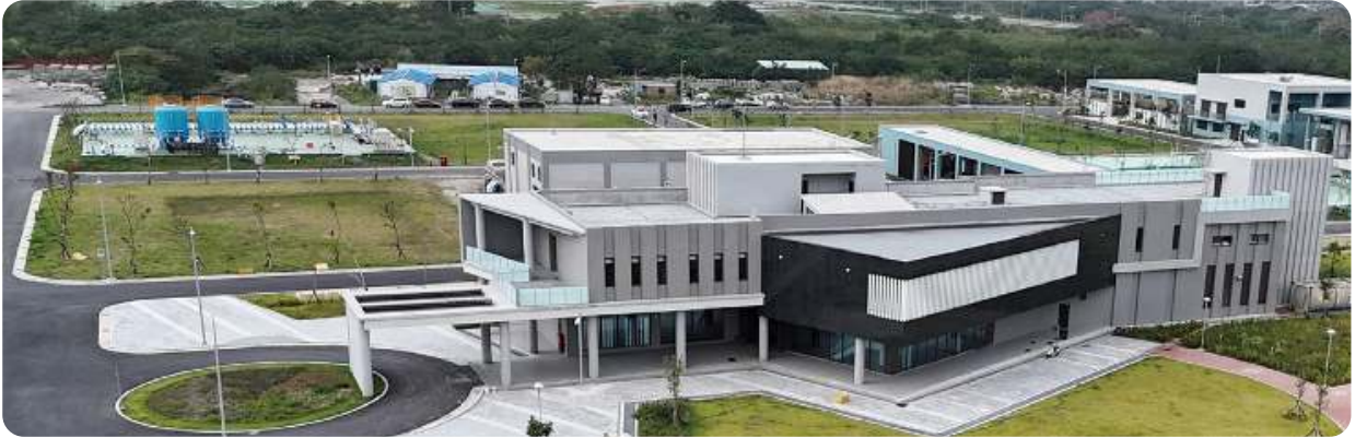
CTSP Erlin Park Water Resource Center
