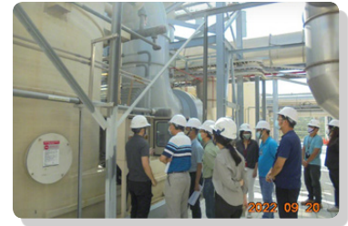
Inspection by experts and scholars of fixed pollution sources
