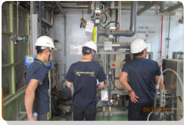
Permit check of water pollution sources
