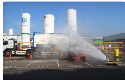
The fire department used water mist to guard the tank car from leaking and stopping drilling
