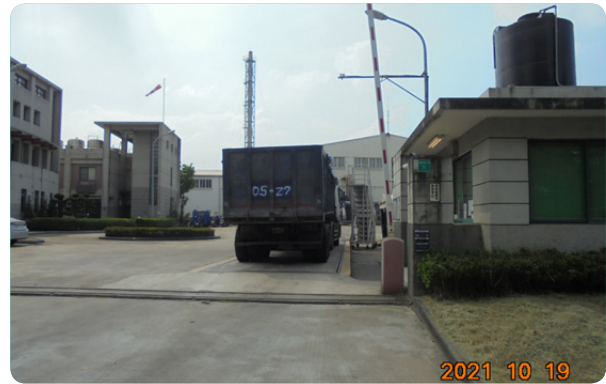
Sewage treatment plant sludge removal truck accompanied by vehicle (Houli)
