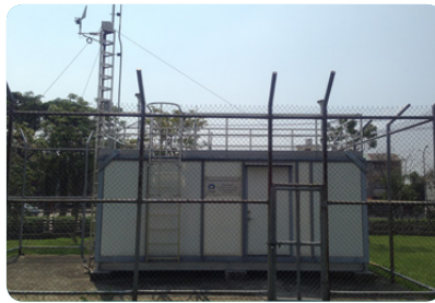
Air Quality Monitoring-Houli Park - Qixing Base General Air Quality Monitoring Station
