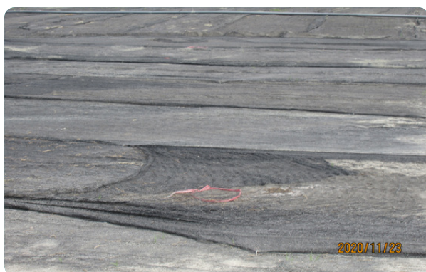
Bare work surface areas are covered with netting to prevent dust
