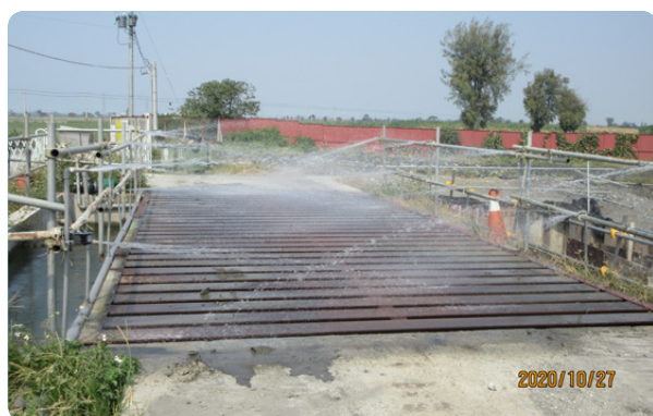
Vehicle washing platform at the entrance and exit of the construction site
